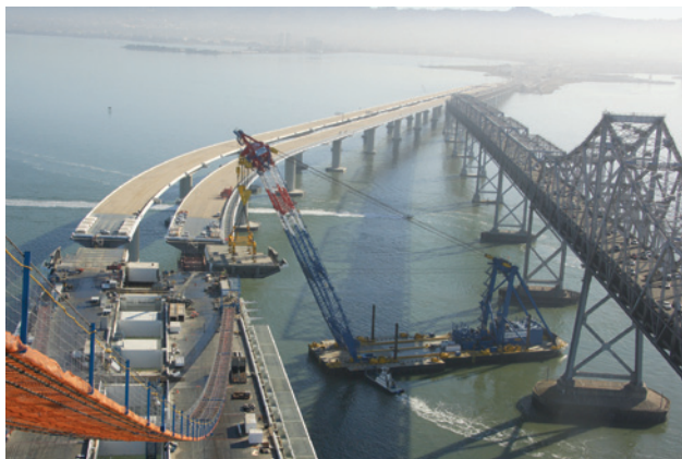
Lifting of a segment of the new Bay Bridge as seen from the new Bay Bridge tower.
