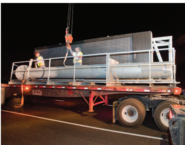
Installation of an overhead changeable message sign along State Route 99.
