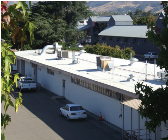
A view of the cool roof on a District 5 building in San Luis Obispo.
