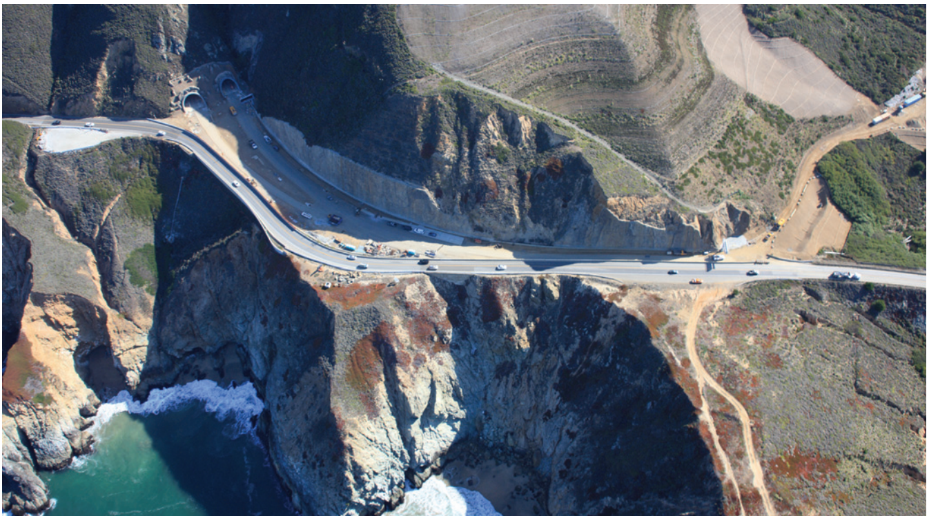
Aerial view of the south portal and roadway of the Devil's Slide Tunnel.
