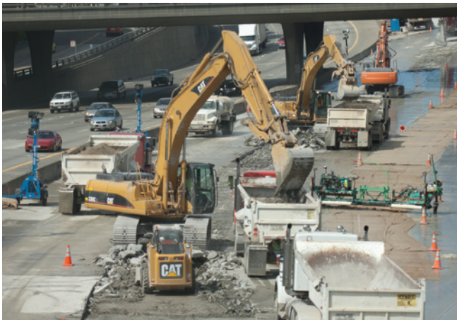
Closure and rehabilitation of I-5 near downtown Sacramento in 2008.
